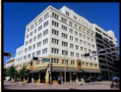
Guaranty Building West Palm Beach, Florida
