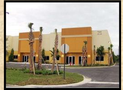
Haverhill Business Park West Palm Beach, Florida
